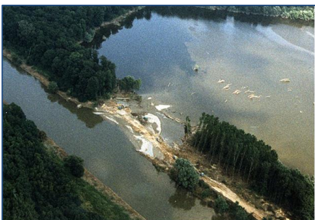
Fig. 1 The collapsed levee at Kvasice on the Morava River
