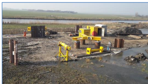
Sheet pile push over tests
